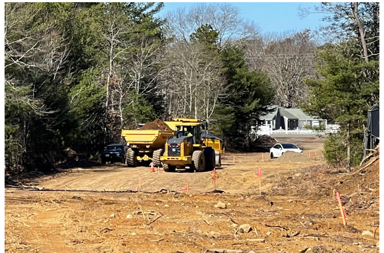
Route 130 Entrance Infrastructure
