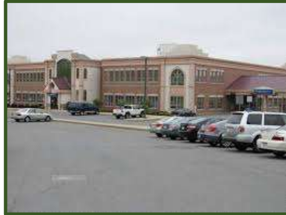
First Federal Savings Bank Swansea, MA
