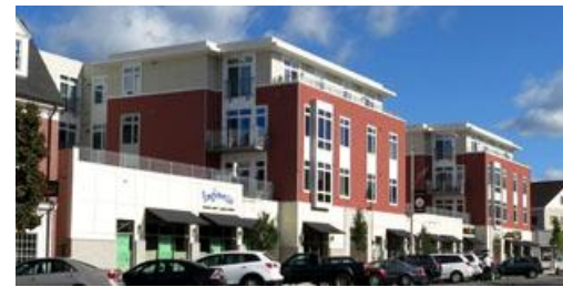
30 Haven, Reading MA includes fifty-three one-and two-bedroom homes and 22,000 SF of retail space on the ground level.
