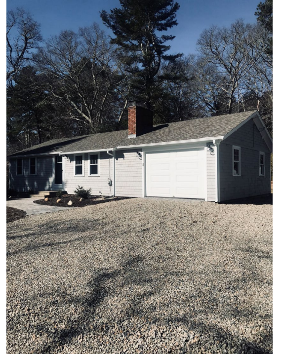
Shore Drive New Construction
