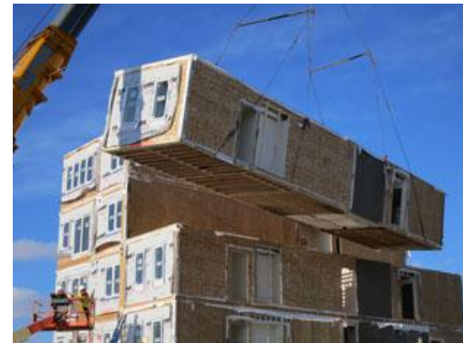
Simultaneous site preparation and modular fabrication compresses construction time. 30 Haven's 108 boxes were set in 3 1/2 weeks.
